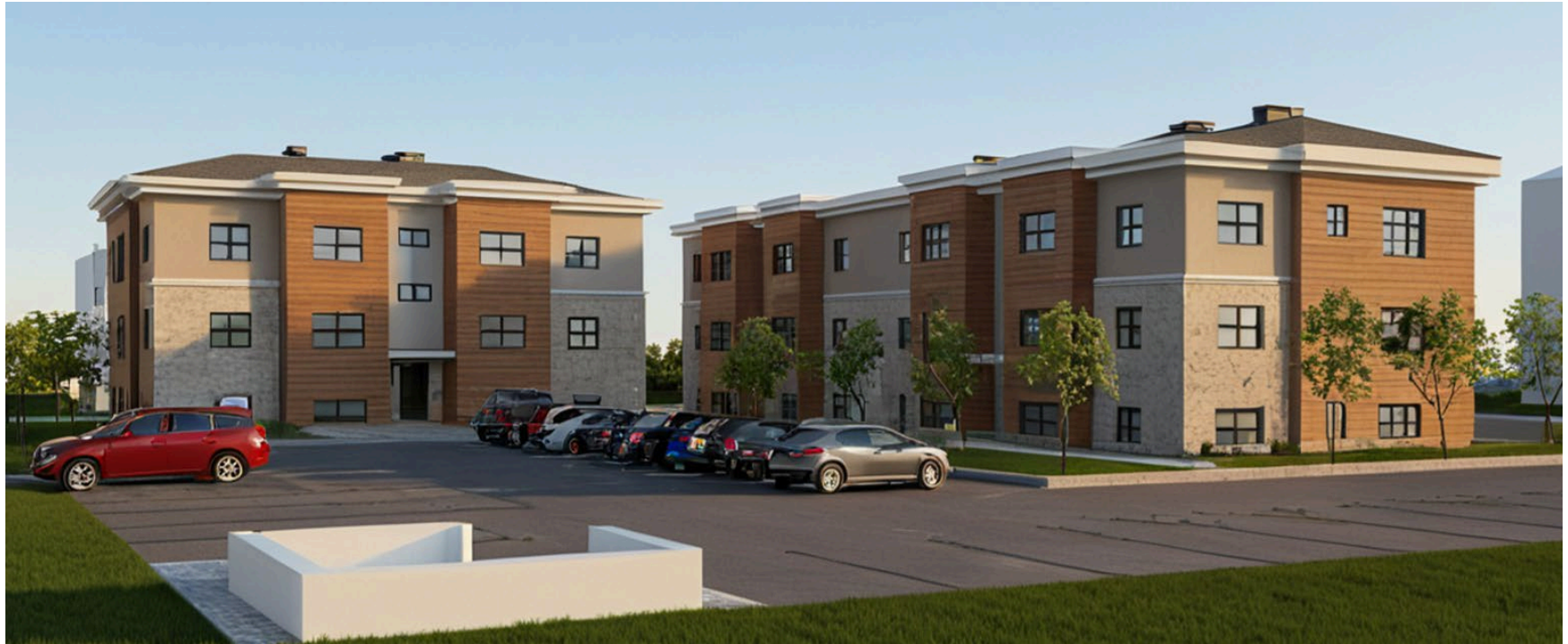
View from parking area
